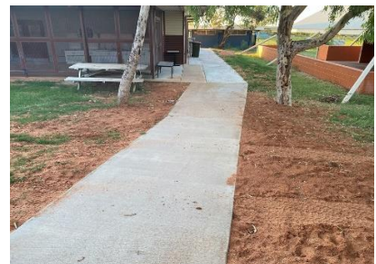
December 2021: RL Build installation of 155 metres of concrete pathways.
